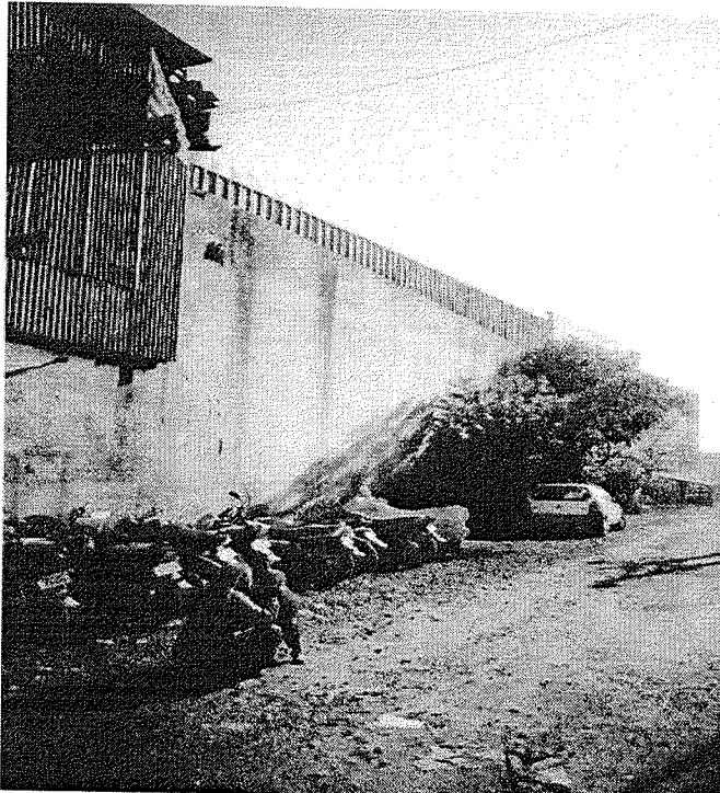
STAFF PARKING IN FRONT ELEVATION OF FACTORY
