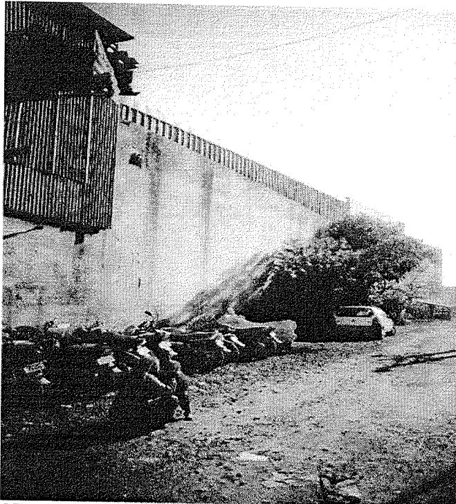
STAFF PARKING IN FRONT ELEVATION OF FACTORY
